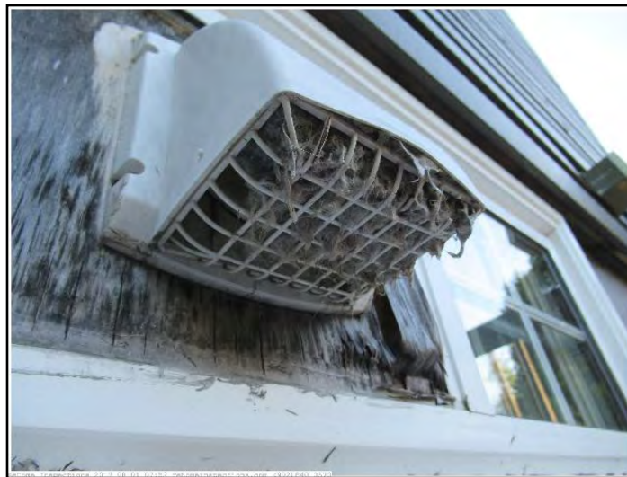
dryer vent screened
