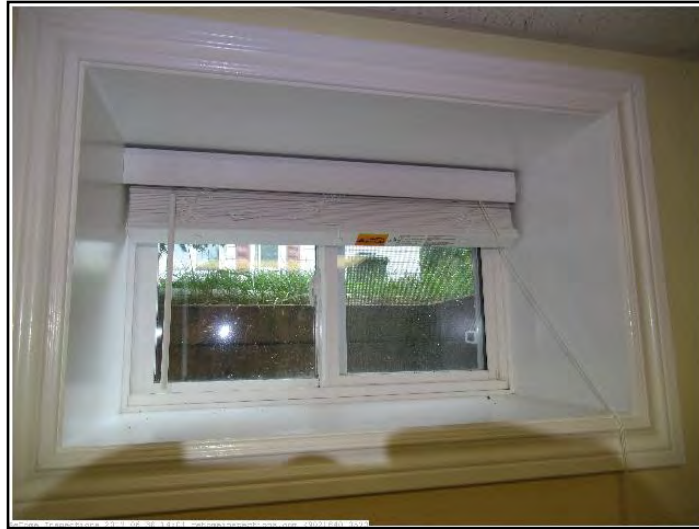
inadequate egress in basement bedroom
