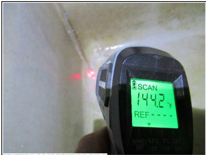
Kitchen sink - HOT!
