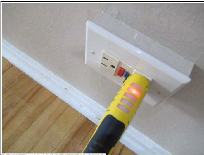
upgraded to GFCI - okay
