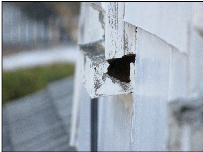
rotted window sill/nosing
