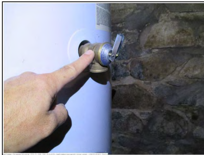
TPRV discharge tube missing
