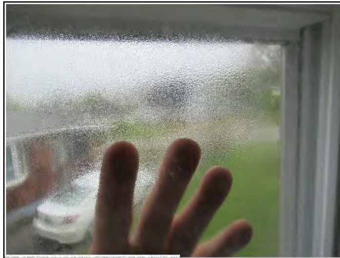
broken window seal
